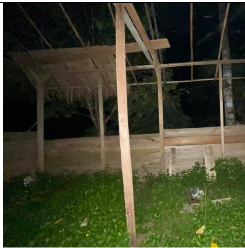
Figure 34: Renovating coffee production house in Senamat Ulu
