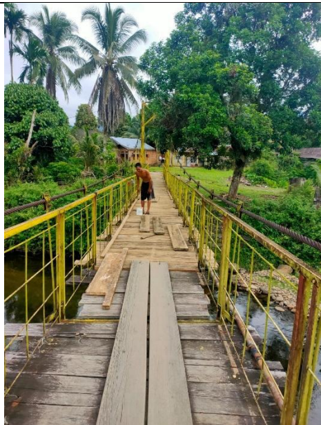
Figure 35: Renovating hanging Bridge in Laman Panjang Village
